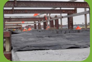
Thermal or heating blankets can be used to thaw ground or to prevent it from freezing. After the pour the same blankets are used to cure the concrete.
