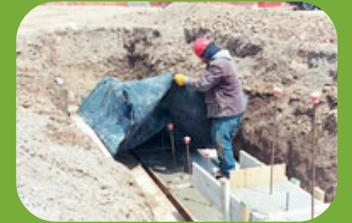
Use a tarp to cover footings and leave formwork in place.
