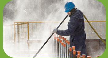
Clearing snow from Formwork using compressed air.
